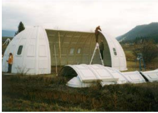
End Pieces Connected Ready to Place Front Panels
