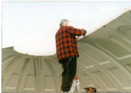
Preparing for the Roof
