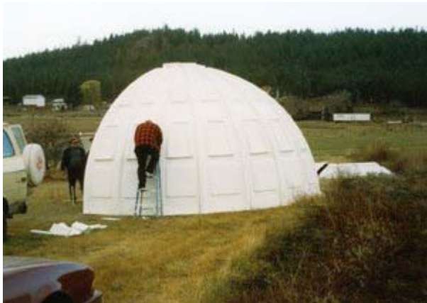
Dome Home Erection Process Getting Started
