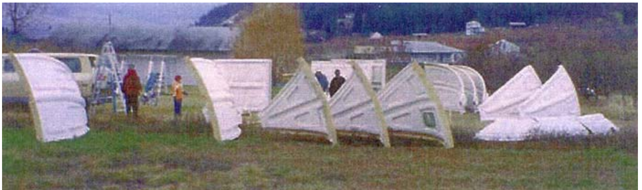
Manufactured Transglobal Dome Home Components On Building Site
