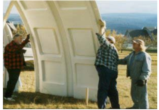
Installing Front Panels and Determining Placing of Door
