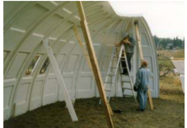
Connecting Back Panels to End Pieces
